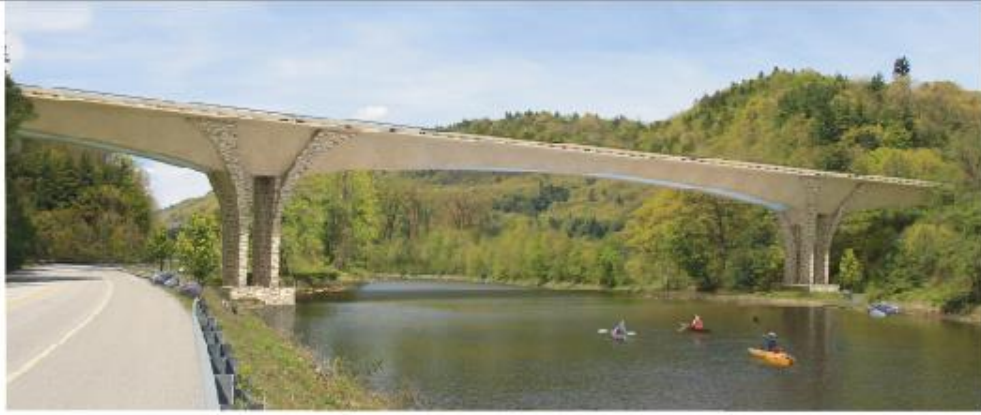
I-91 Bridge view from Route 30 looking north
