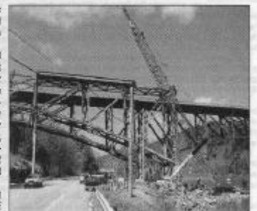
Construction on the I-91 bridge on April 9.
