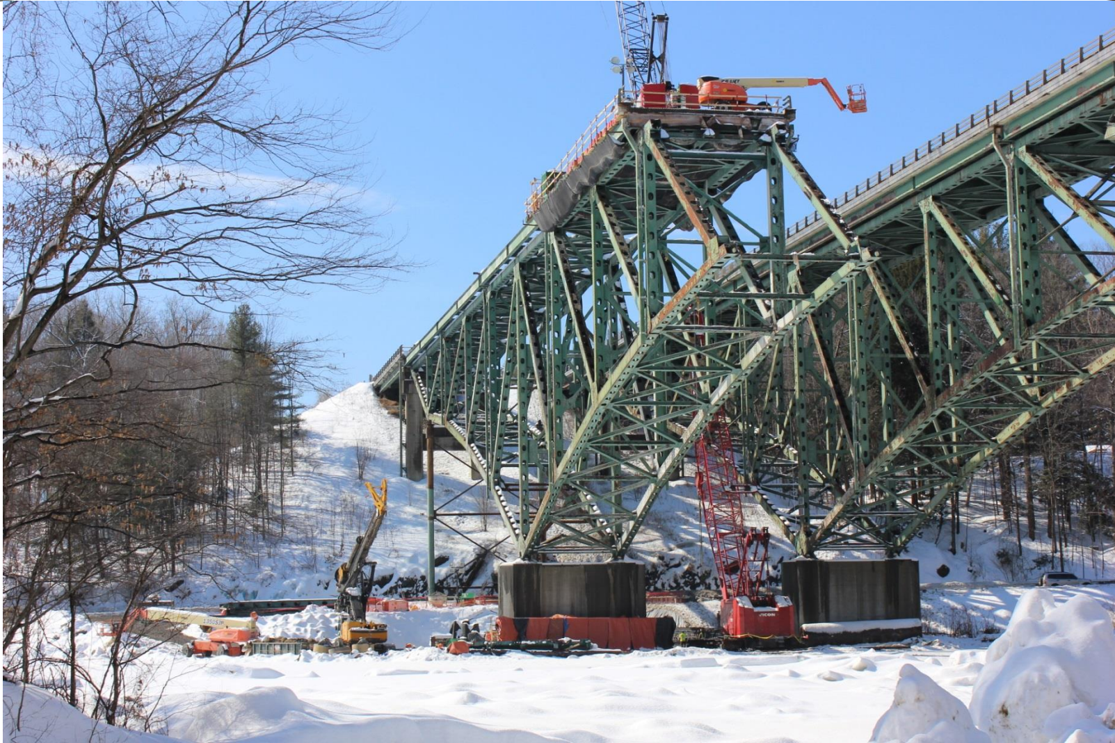
Demolition of Bridge 8S and 9S
